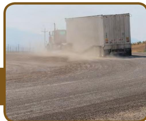
*A truck kicks up a substantial amount of dust on a road that has not been treated with any kind of dust suppressant.*
