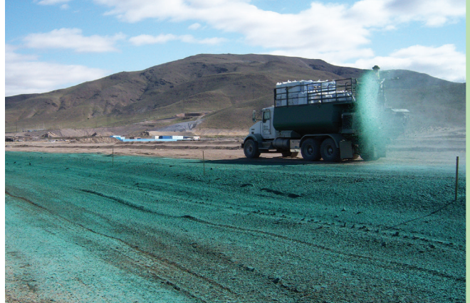
Photos courtesy of Apex Erosion Control (top) and Mark Seeding (bottom)
