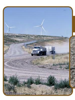
A truck kicks up a substantial amount of dust on a road that has not been treated with any kind of dust suppressant.
